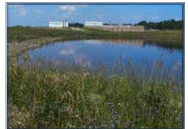
*Holding pond for control of runoff.*
